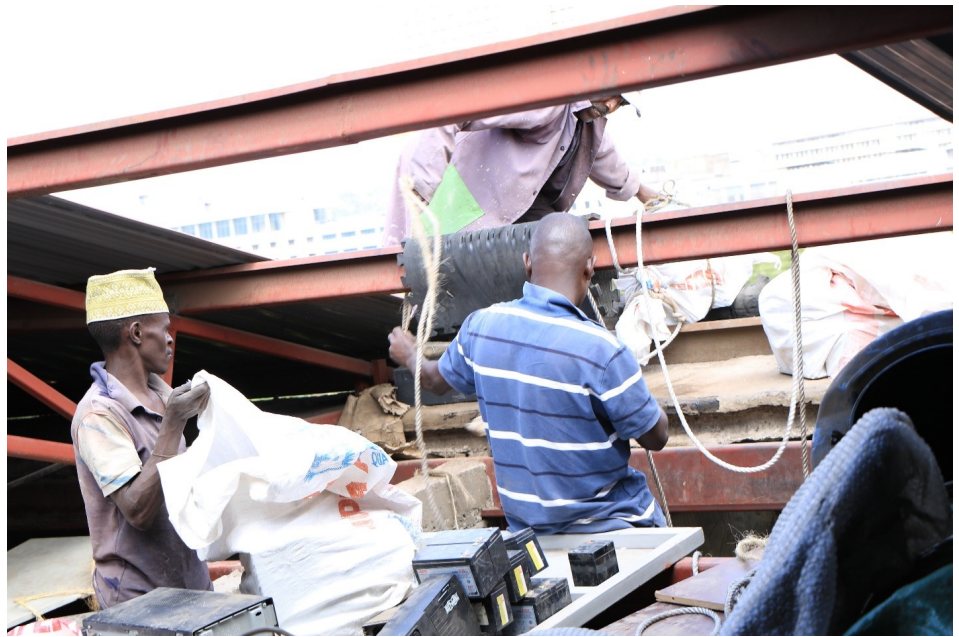
Workers on the construction site on 5 th floor of Commission House
